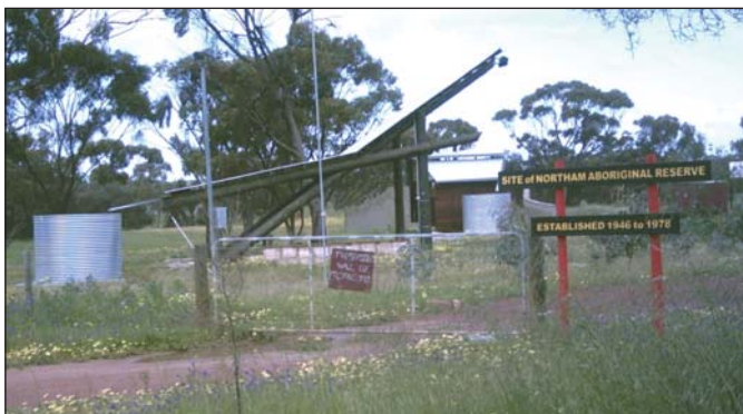
Figure 1: Northam Reserve - New buildings
